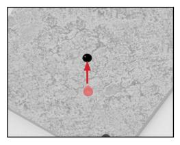
11. Insert the silicone plug into the fixture opening to prepare for finishing. The fixture must remain off for the remainder of the installation.
