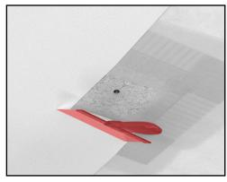
14. Apply the subsequent coat of plaster to level out the board with the existing drywall finish.
