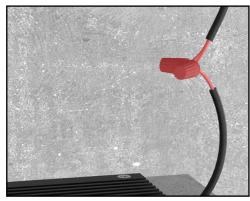
8. Feed low voltage wiring to the bracket and lift the fixture board assembly to the low voltage electrical connection and make the connection.
