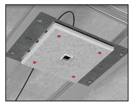
**7.** Secure the board to the drywall bracket using the provided screws.
