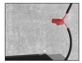
**5.** Feed **low voltage** wiring to the bracket and lift the fixture board assembly to the **low voltage** electrical connection and make the connection.
