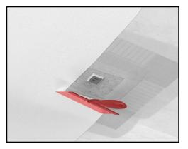
**12.** Apply the subsequent coat of plaster to level out the board with the existing drywall finish.
