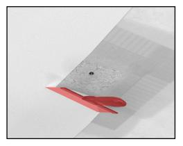
11. Apply the subsequent coats of plaster to the ceiling, making sure again to minimize the amount of plaster applied to the fixture board assembly.
