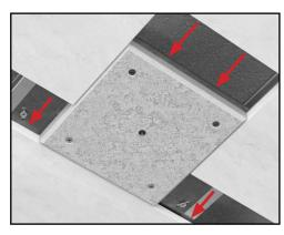
8. Cut and install the drywall around the fixture, ensuring that the fixture board assembly is flush with the surrounding drywall. This will allow a finish of one eight inch of plaster around the board.
