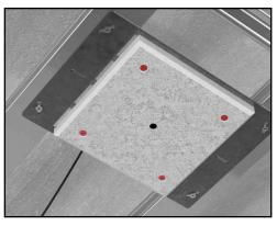
6. Secure the board to the drywall bracket using the provided screws.
