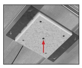
7. Insert the silicone plug into the fixture opening to prepare for finishing. The fixture must remain off for the remainder of the installation.
