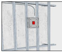
**1.** Identify the desired fixture location and raise the bracket to the framing.
