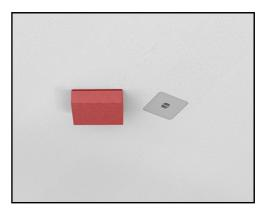
**16.** Wait until the surface has fully dried, and sand the plastered ceiling to match the surrounding level of drywall.
