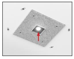
**10.** Insert the fixture board assembly into the cutout. Test the fixture is fully operational. Do not move on to the next step until the fixture is operational.
