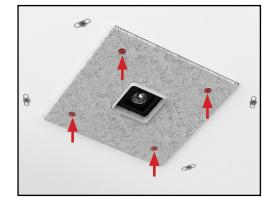
**11.** Secure the board to the drywall bracket using the provided screws.
